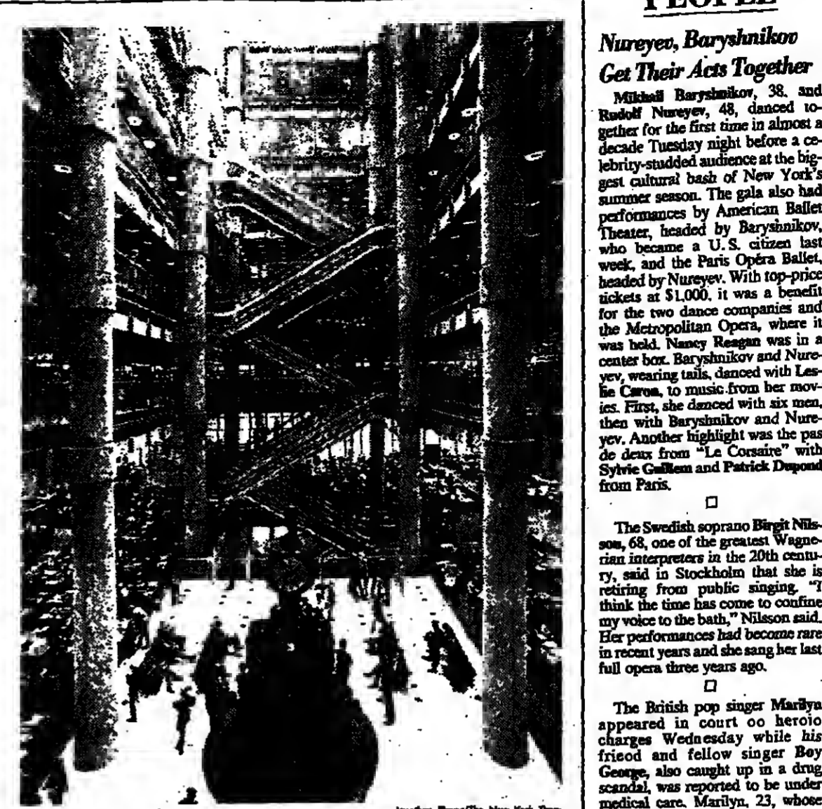
View of the floor and galleries at the new Lloyd's Building.
